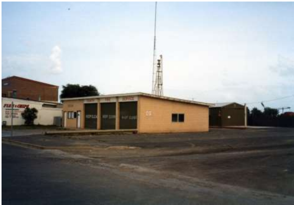
Alexandrina Library Collection, by Walter Pretty – Goolwa Country Fire Service and St John Ambulance Depot, corner Cadell & Crocker Streets, Goolwa. 29 March 1987.
